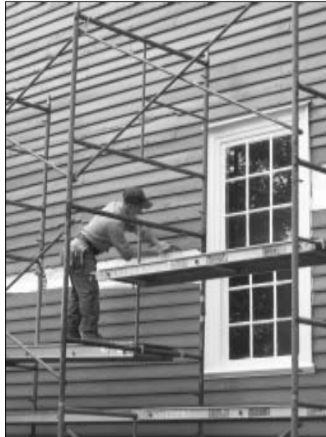
Tom Burdette replaces Ellwood siding.
